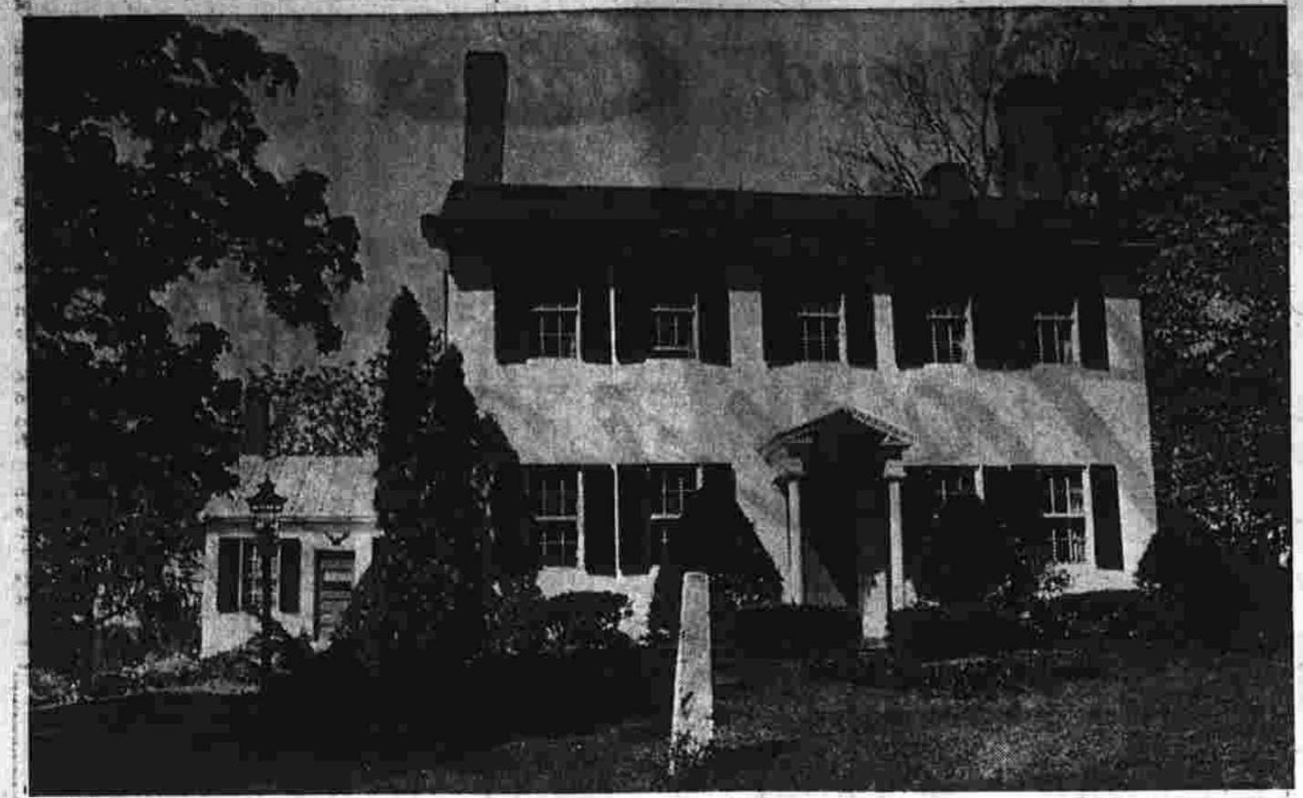
The Gov. John S. Peters house, built in 1806, with brick made in town, is one of the homes on the tour.
